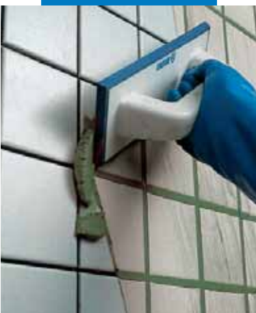
Spreading Ultracolor Plus on a wall with a rubber trowel
