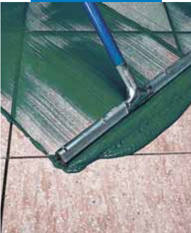
Spreading Ultracolor Plus on a floor with a rubber sponge
