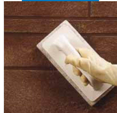
Cleaning the joints with Scotch-Brite® (product partially set)
