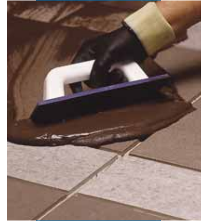
Spreading Ultracolor Plus on a floor with a rubber trowel
