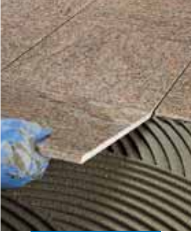
Installation of pre-glossed marble on floors
