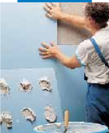
Laying polystyrene foam slabs with Keraflex white
