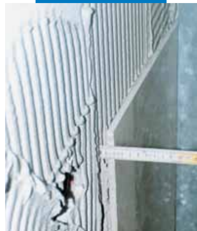
Thickly applied porcelain tiles on a wall
