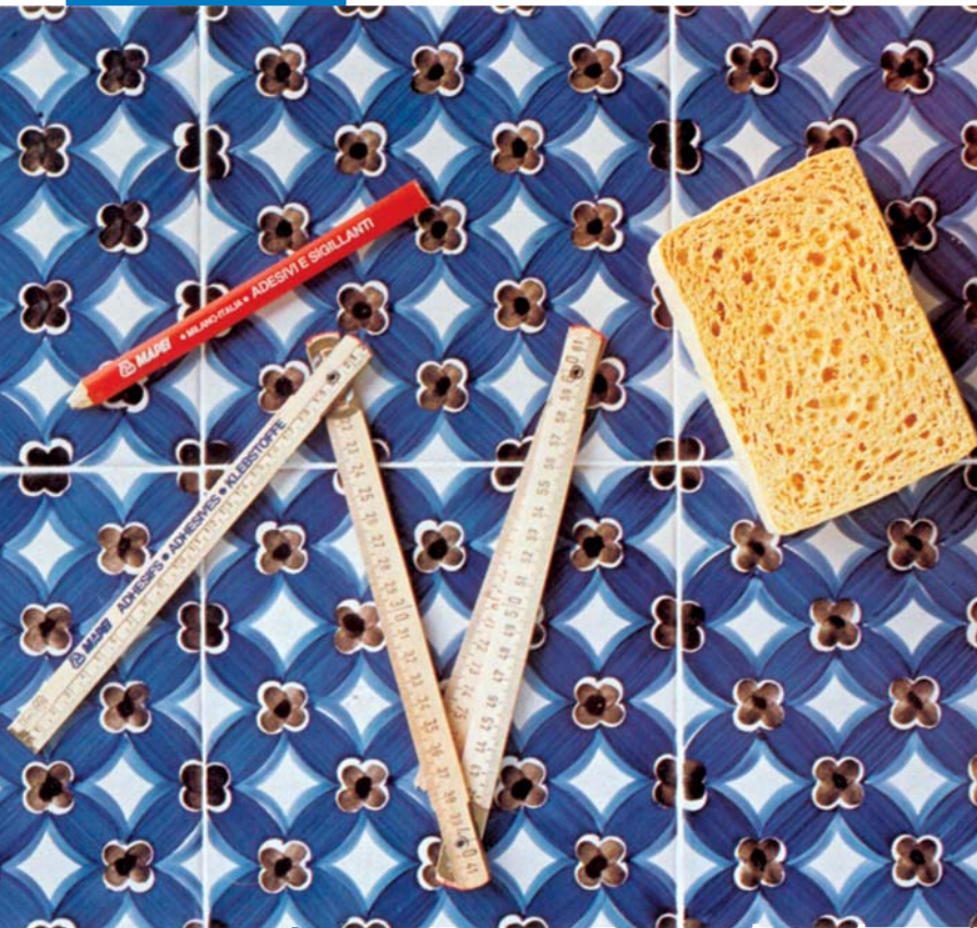
Grouting tight-joint tiles
