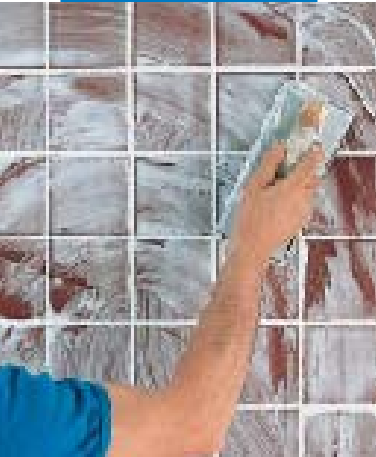
Spreading with a rubber float
