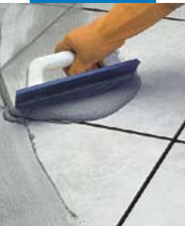
Grouting a ceramic tile floor with a sponge trowel
