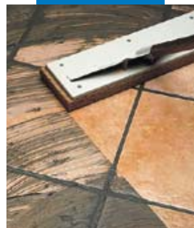
Cleaning a single-fired tile floor with a sponge brush
