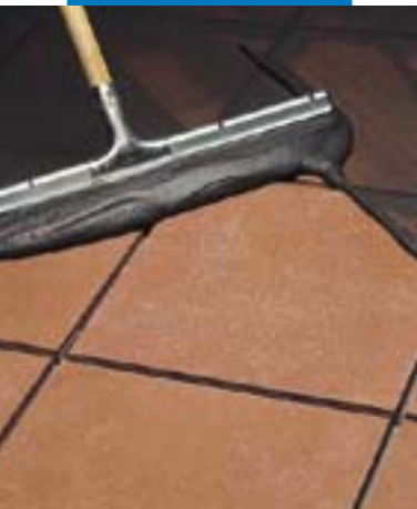
Grouting a terracotta tile floor with a rubber float
