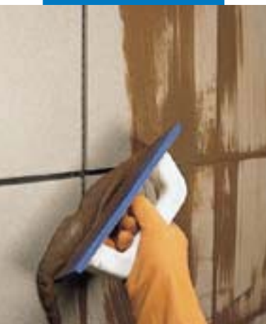
Grouting an external wall with a trowel
