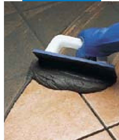
Grouting single-fired tile with a trowel
