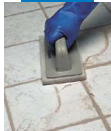
Finishing with a Scotch-Brite® pad
