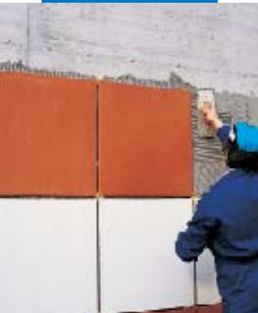
Fixing large size tiles with Kerabond + Isolastic
