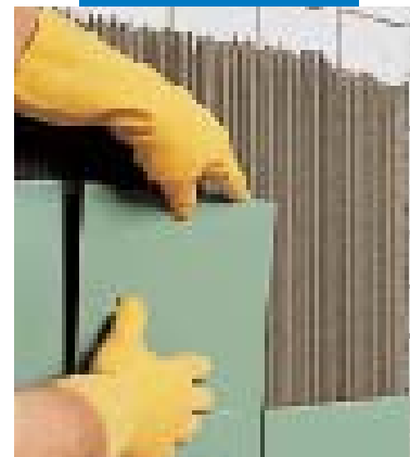
Laying over old tiles
