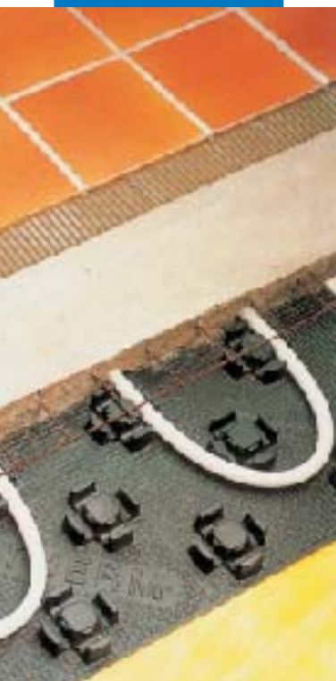
Laying over an underfloor heating installation
