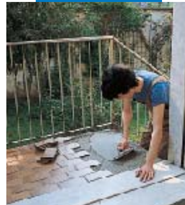
Waterproofing levelling and laying with Kerabond + Isolastic
