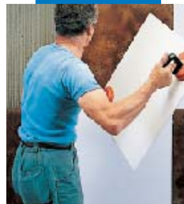
Laying KERAION on a wall
