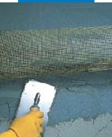
Waterproofing with Mapelastik reinforced with Fibreglass mesh
