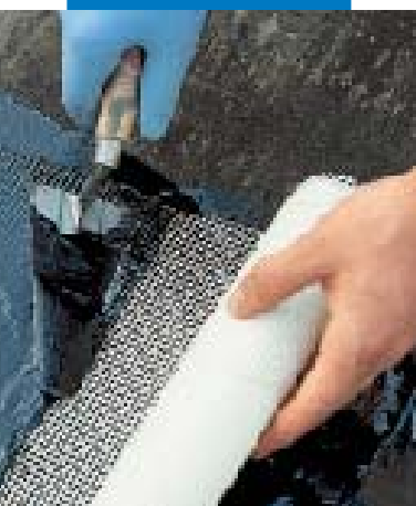
Repairing cracks with Plastisol 1 reinforced with Fibreglass mesh
